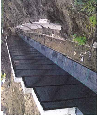
Foundation waterproofing
