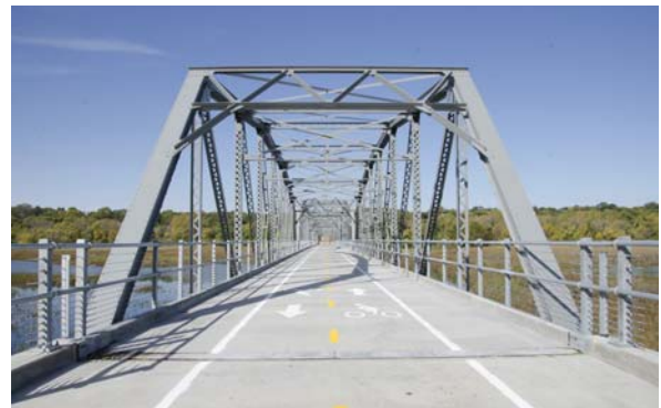
Completed Old Cedar Avenue Bridge
