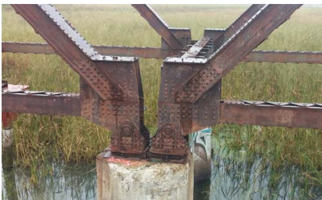
Bearing Reconstruction – Old Cedar Bridge
