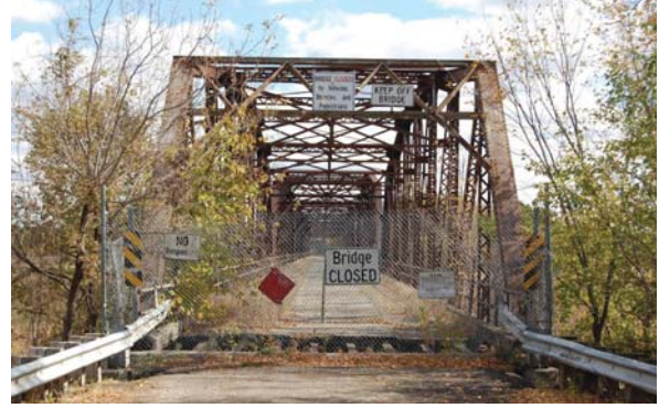
Photo of existing bridge
