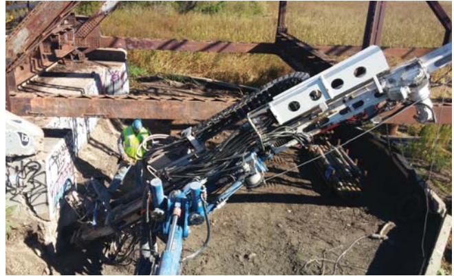
Abutment Stabilization Anchor Installation – Old Cedar Bridge
