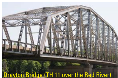
Drayton Bridge (TH 11 over the Red River)
