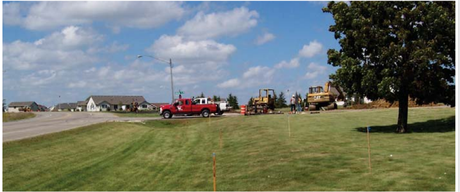
Summarized defects identified in the I/I investigations and lined the sewer at strategic points to reduce infiltration and restore the structural integrity of the pipe.
