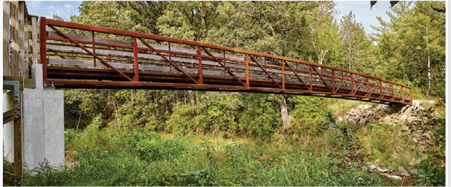
WHKS worked with FEMA and other agencies for disaster relief funding to replace the structure.
