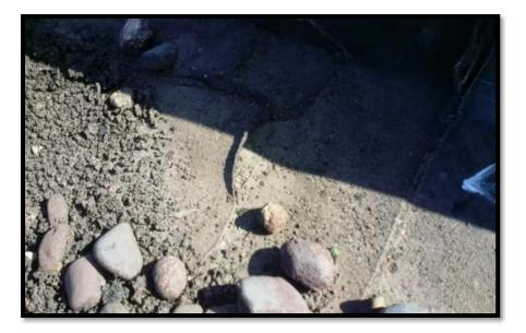
5) Defect: Membrane Flashing Unbonded Repair: Install EPDM Patch Roof Location: 5
