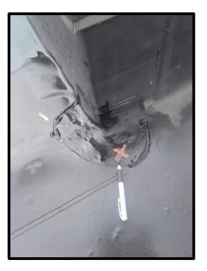
Defect: Membrane Flashing Hole Repair: Install EPDM Patch Roof Location: 1 Units: 2 Repair Type: Immediate Repair Cost: \$353.00
