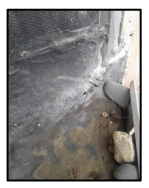
6) **Defect:** Deteriorated Pitch Pans **Repair:** Install New Pitch Pan Filler
