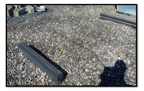
4) Defect: Membrane Flashing Unbonded Repair: Install EPDM Patch Roof Location: 2
