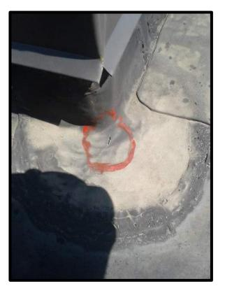
5) Defect: Membrane Flashing Unbonded Repair: Install EPDM Patch Roof Location: 2 Units: 2 Repair Type: Immediate Repair Cost: \$353.00
