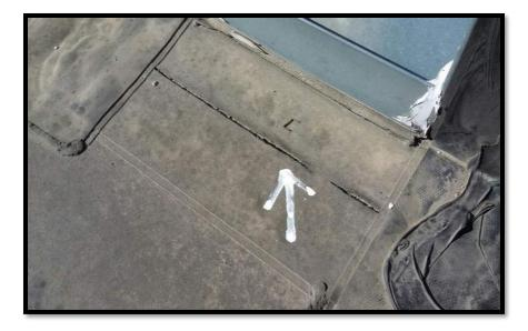
Defect: Membrane Flashing Unbonded Repair: Install EPDM Patch Roof Location: 1 & 2 Units: 9 Repair Type: Immediate Repair Cost: \$700.00
