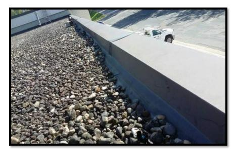
Defect: Obsolete Equipment Repair: Remove Sleepers and Patch Area Roof Location: 2 Units: 2 Repair Type: Life Extension Repair Price: \$1,785.00
