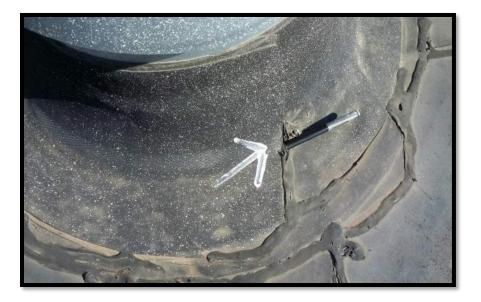
Defect: Perimeter Membrane Securement Defective Repair: Reflash Perimeter Roof Location: 1 Units: 70 Ln.Ft. Repair Type: Life Extension Repair Price: \$4,694.00
