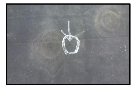
4) Defect: Membrane Flashing Hole Repair: Install EPDM Patch Roof Location: 2
