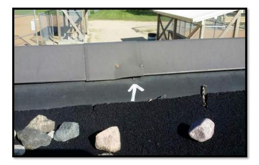
2) **Defect:** Perimeter Membrane Securement Defective **Repair:** Reflash Perimeter
