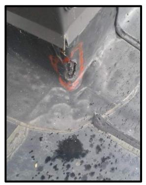
4) Defect: Membrane Flashing Hole Repair: Install EPDM Patch Roof Location: 1
