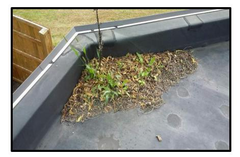
3) Defect: Membrane Hole Repair: Install EPDM Patch Roof Location: 1 Units: 1 Repair Type: Immediate Repair Price: \$229.00
