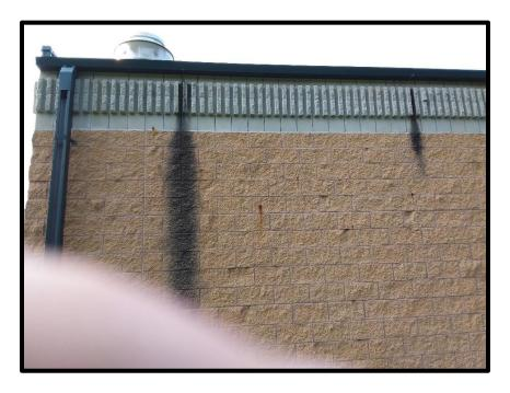
4) **Defect:** Membrane Flashing Unbonded
