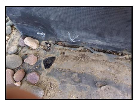
2) **Defect:** Membrane Flashing Unbonded
