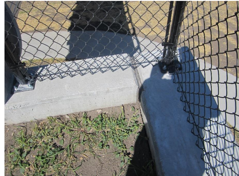
Chain Link Fence Mounted on MSE Wall Coping
