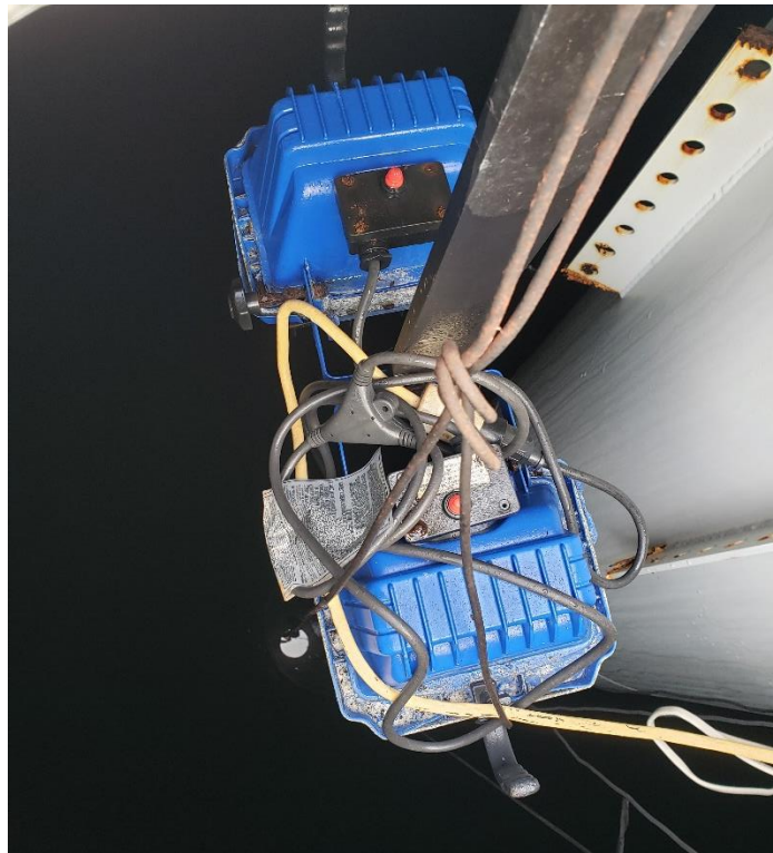
EXISTING INTERIOR LIGHTING AND CAMERA TO BE REMOVED
