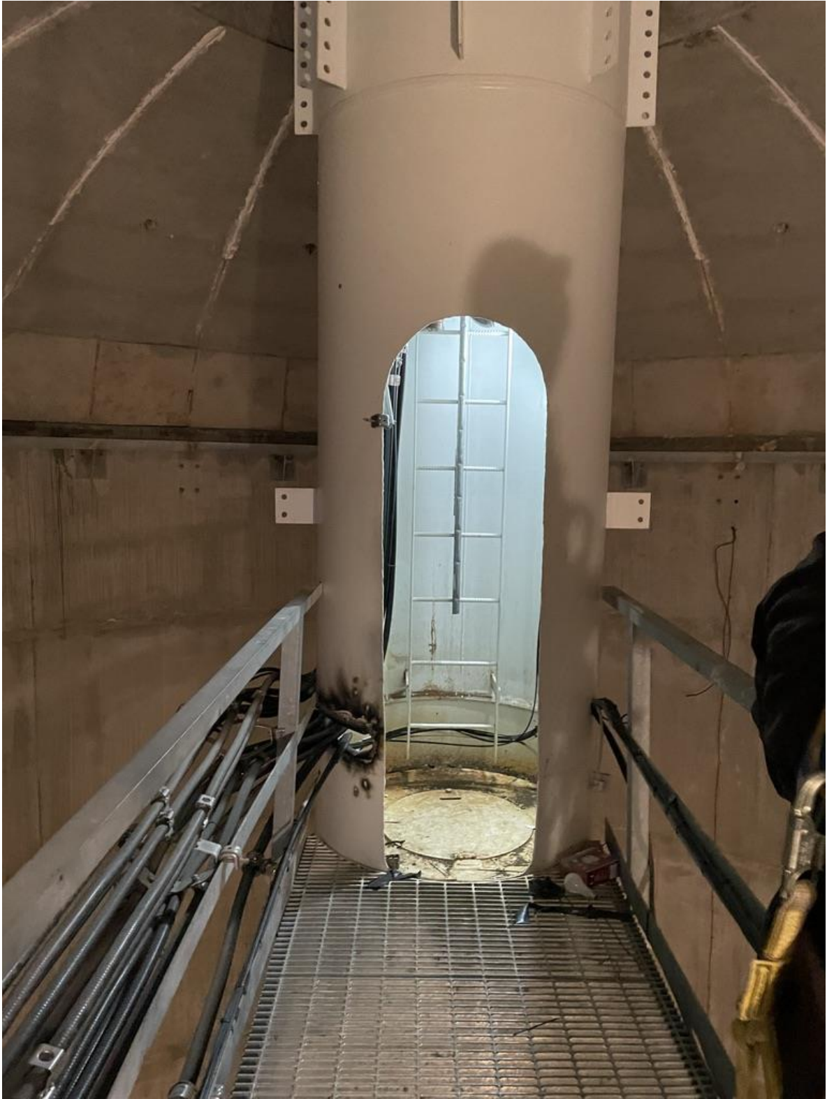
EXISTING CATWALK ENTRANCE TO ACCESS TUBE AT TOP OF PEDESTAL
