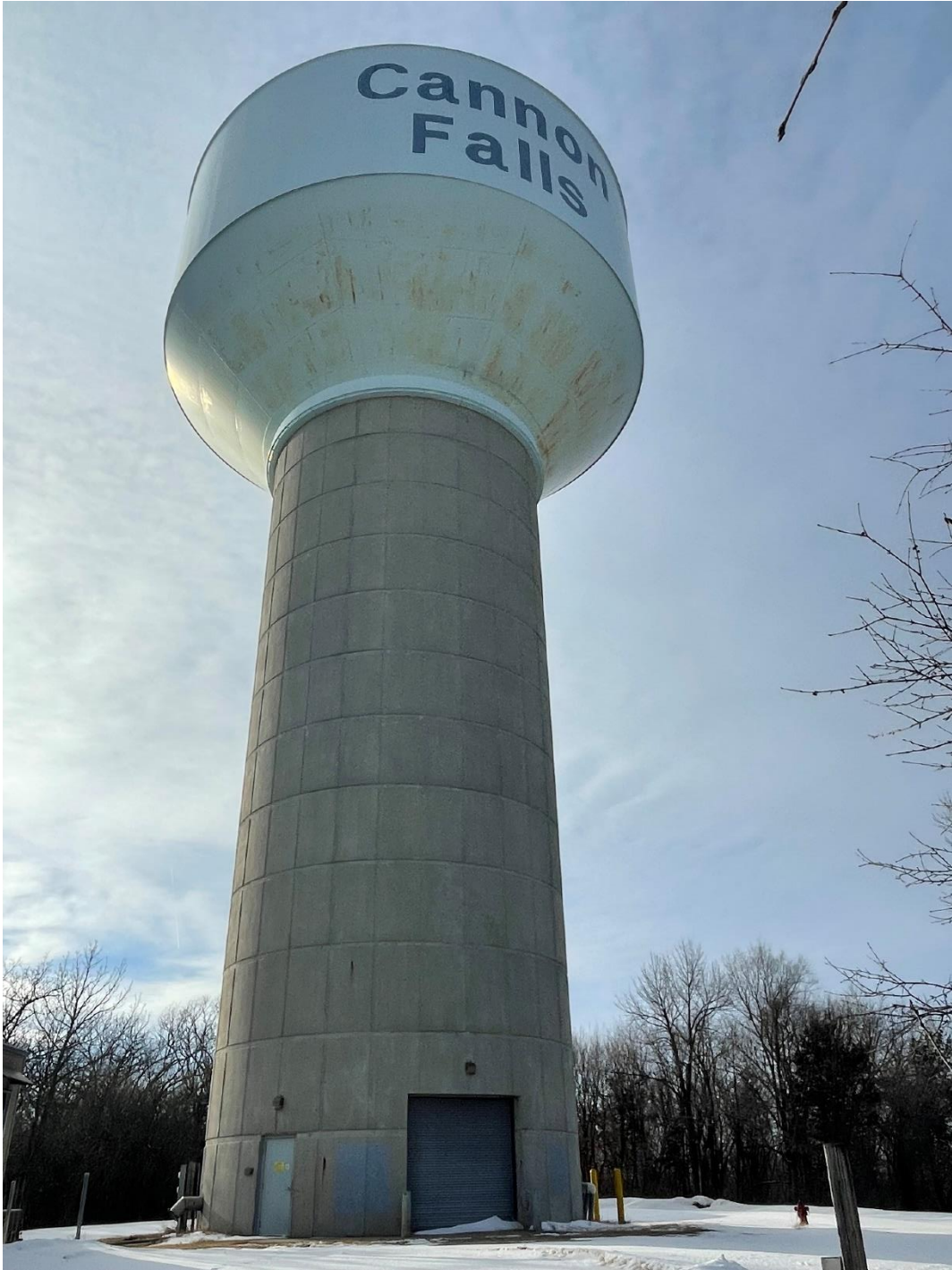
EXISTING WATER TOWER
