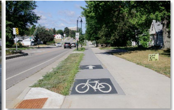
▲ Curb separated directional (one way) cycle track adjacent to sidewalk. (Richfield, MN)
