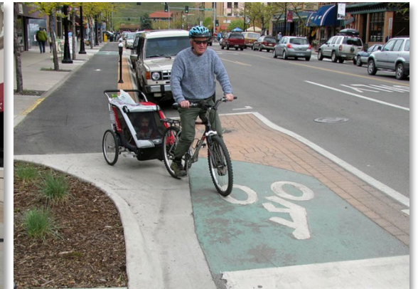
▲ Curb separated cycle track along a downtown Main Street. (Missoula, MT)
