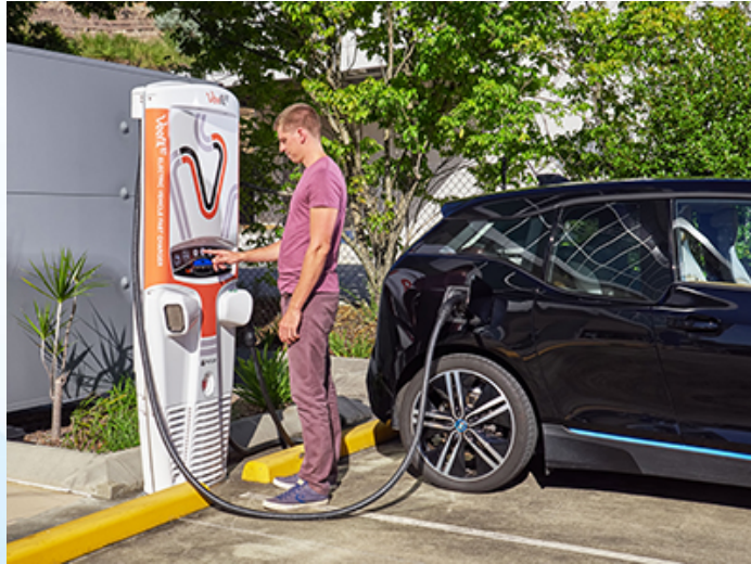
50kW Fast Charger 480v 3P
