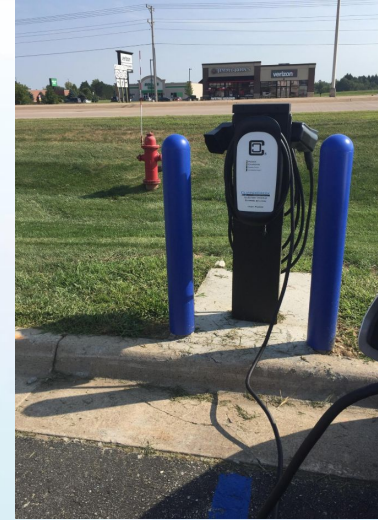
ZEFNET Level 2 Dualhead Charger 2 X 13kW, 240v 1P
